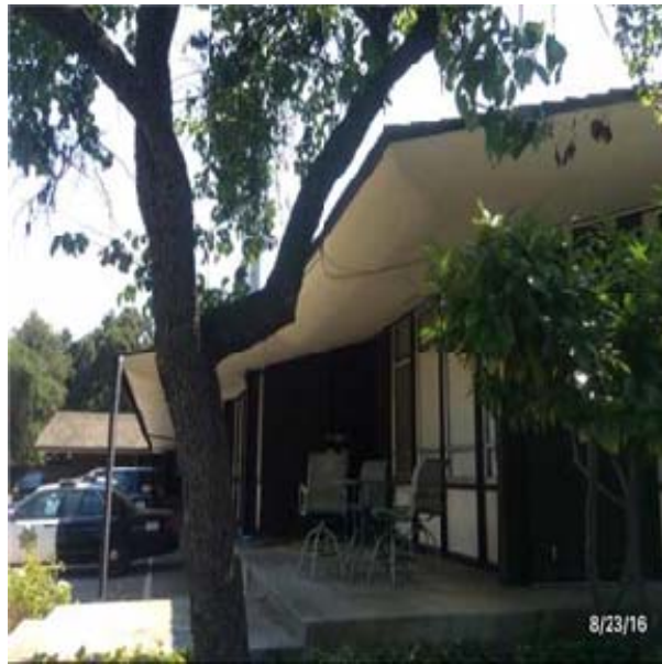
B2021 Windows:- View of Aluminum Window Units - Casement, Double Hung, Vent or Sliding
