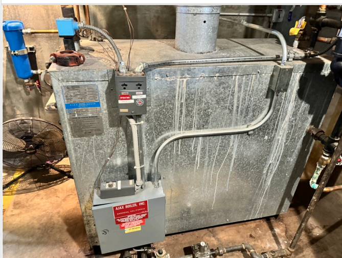
41. Gas-fired boiler
