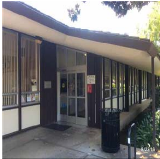
B2031 Glazed Doors & Entrances:- View of Storefronts - Glazed Aluminum Framed with Sliding Door Panels
