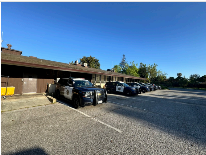
9. Building exterior, paved parking
