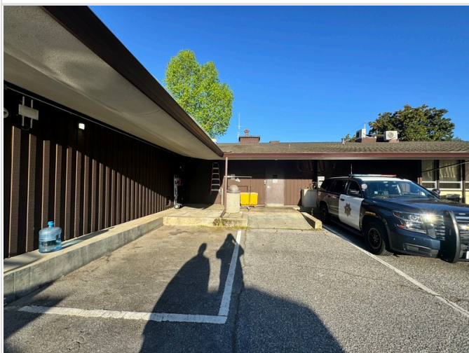
5. Building exterior, paved parking
