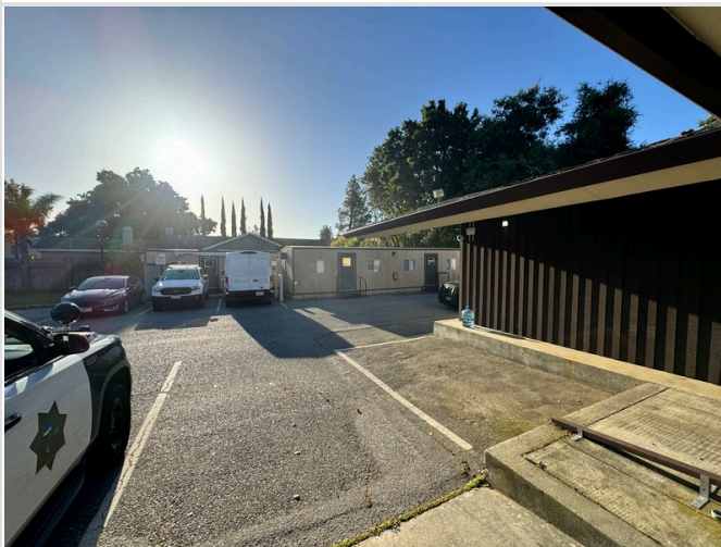
10. Building exterior, paved parking
