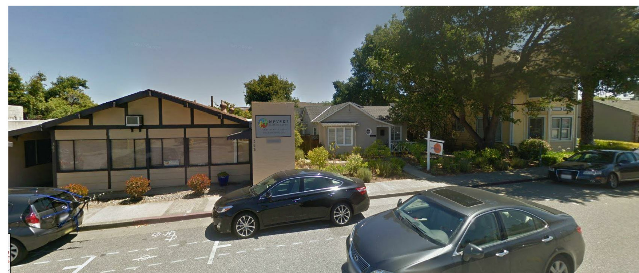
5 - OVERLOOKING FROM THE SITE TOWARDS EAST
