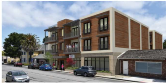
385, 387 & 389 1ST STREET (IN CONSTRUCTION) 4
