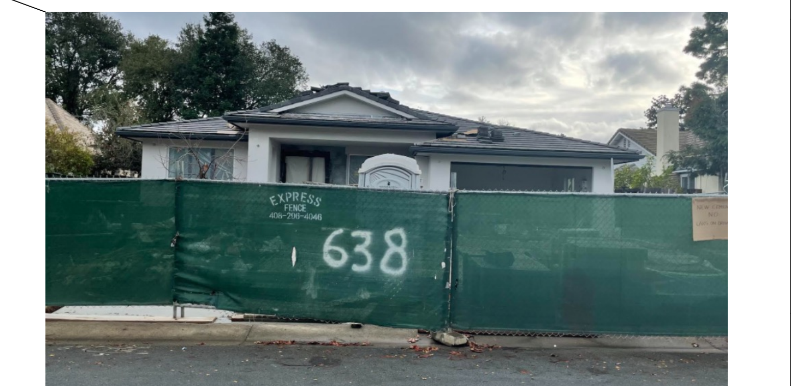
638 BENVENUE AVE (IN CONSTRUCTION) 1-STORY HOUSE
