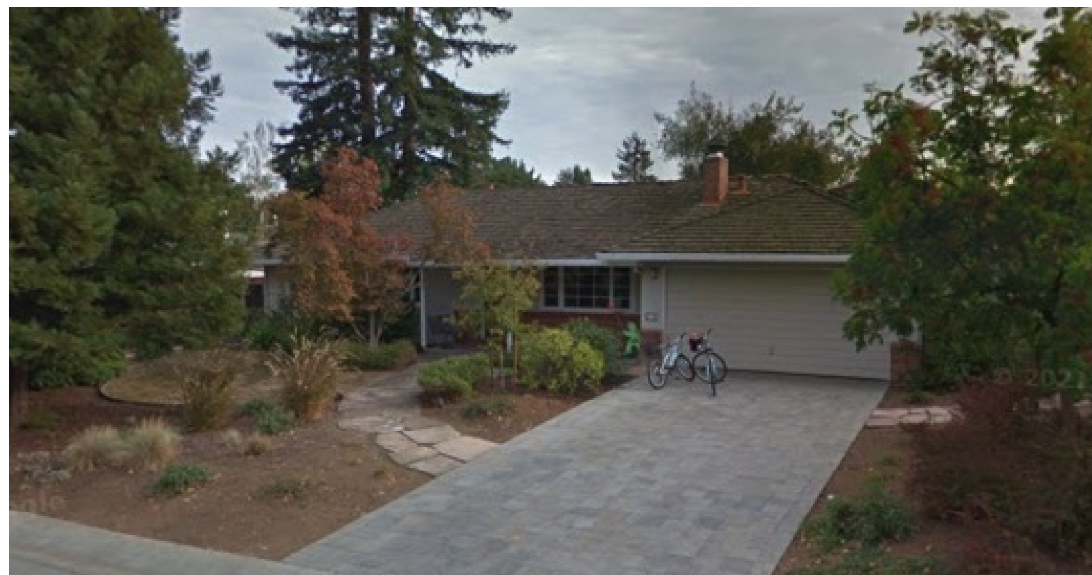
618 BENVENUE AVE 1-STORY HOUSE
