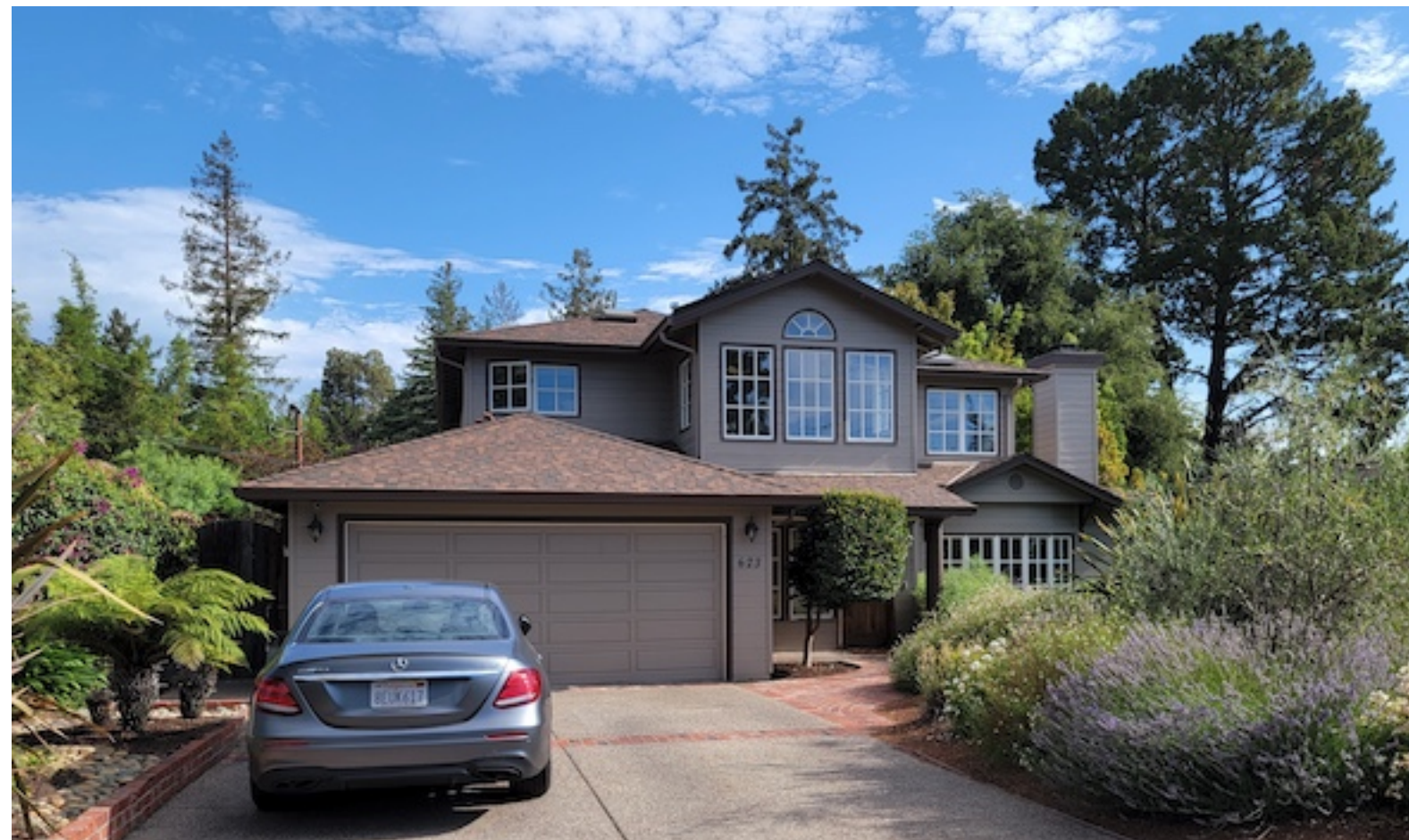
623 BENVENUE AVE 2-STORY HOUSE
