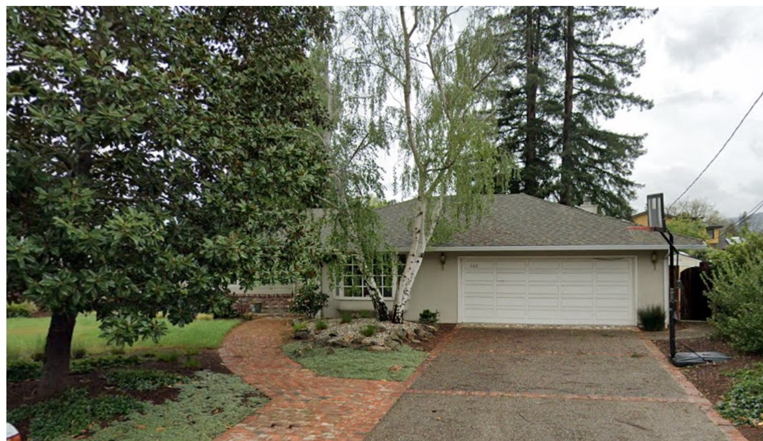
622 BENVENUE AVE 1-STORY HOUSE
