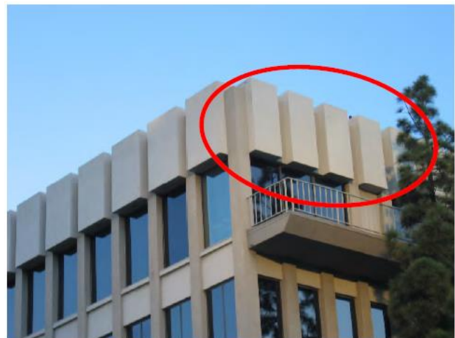
Figure 1: This well-concealed wireless telecommunications facility has its antennas architecturally integrated into the building.
