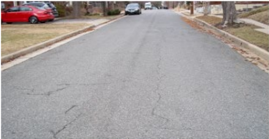
Pavement Condition 71 – 85 (Very Good)
