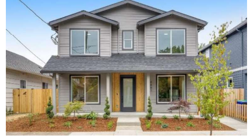
Figure 12. A Newly Built Fourplex in Portland, OR
