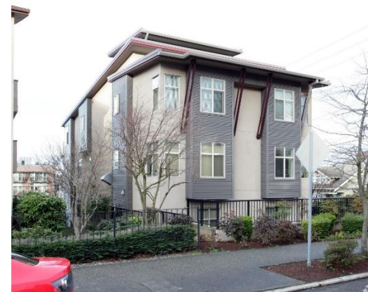
Figure 15. A Fiveplex in the Eastlake Neighborhood of Seattle, WA
