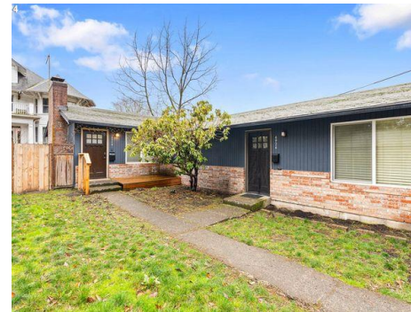
Figure 5. A Single-Story Side-by-Side Duplex in Portland, OR (Source: Zillow ( Link )).
