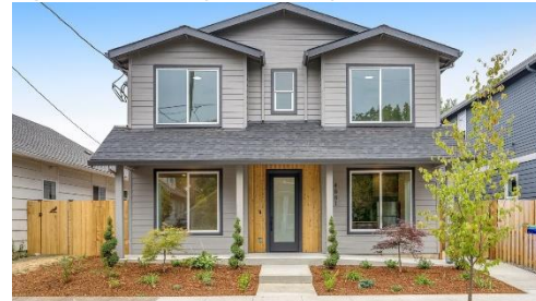
Figure 12. A Newly Built Fourplex in Portland, OR
