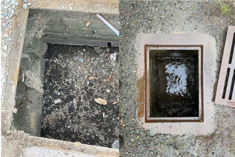
Photo: Typical City catch basin before and after cleaning
