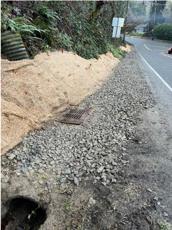
Photo 3: Stabilized site following installation of erosion controls by City of Shoreline Building Department
