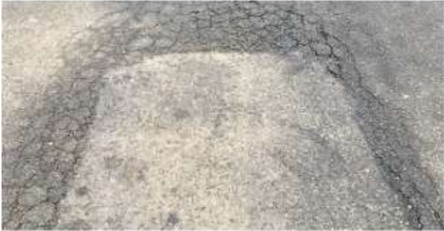
Pavement Condition 0 – 10 (Failed)
