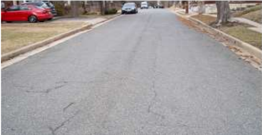
Pavement Condition 71 – 85 (Very Good)
