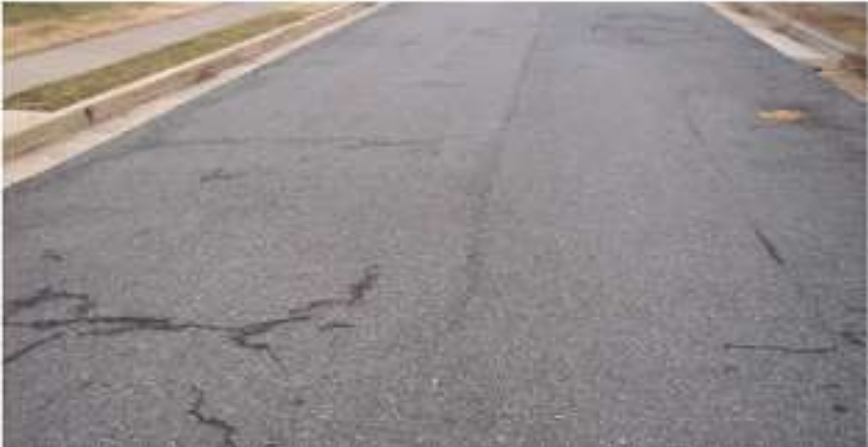
Pavement Condition 71 – 85 (Very Good)
