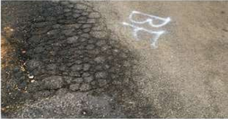
Pavement Condition 0 – 10 (Failed)
