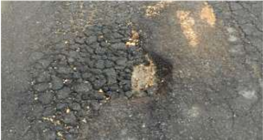
Pavement Condition 0 – 10 (Failed)
