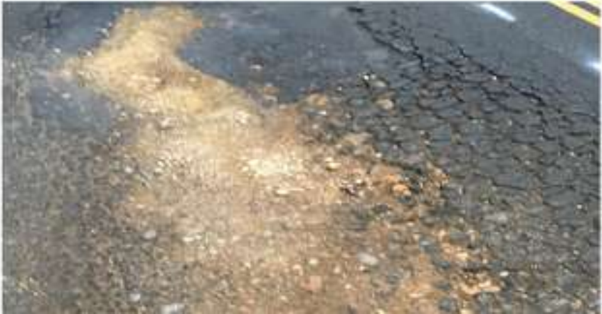
Pavement Condition 0 – 10 (Failed)
