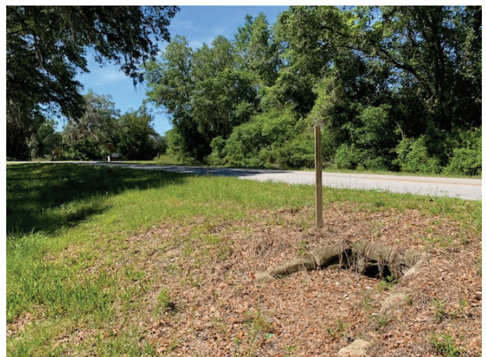
Typical Cross Drain End Treatment
