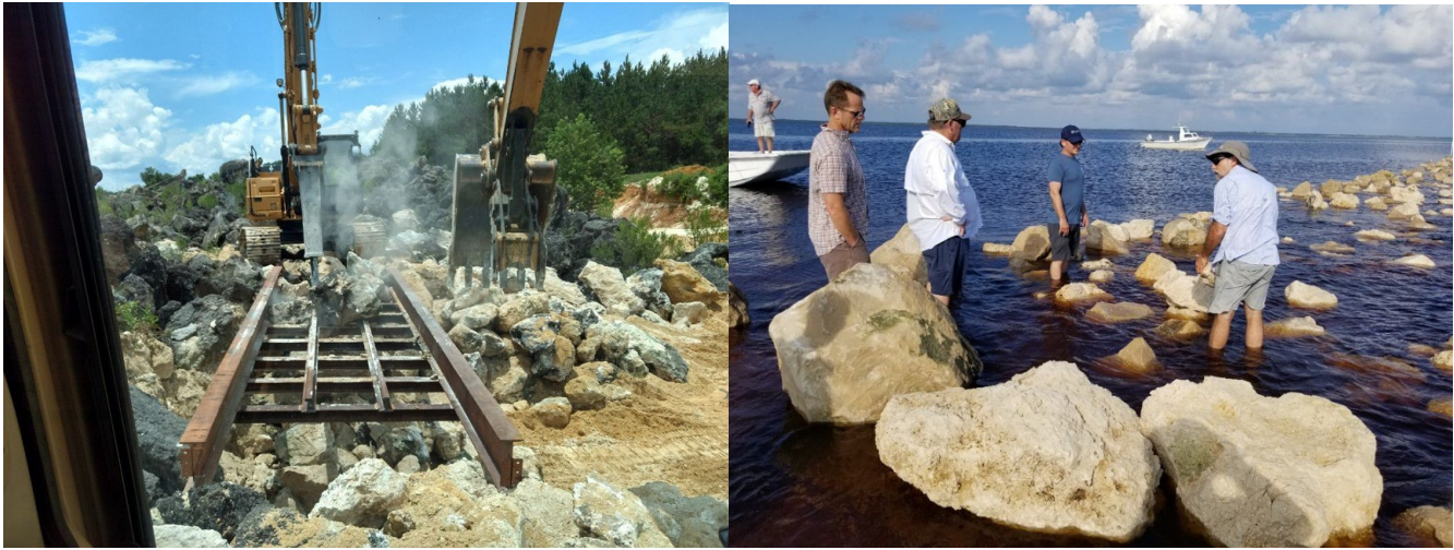
Figure 9. LCR was restored using dolomite limestone from a quarry near Branford, Florida. The top left picture shows the rocks being broken in the quarry. The broken rocks were then trucked to Suwannee, Florida, loaded onto a barge, and then placed on the degraded reef following our construction specifications. The Lone Cabbage project used a mix of large and small rocks as seen in the bottom photo. Our proposed work will use smaller rocks that can be transported by commercial oyster harvesters in skiffs to restore shallow oyster reefs that cannot be restored by barge.
