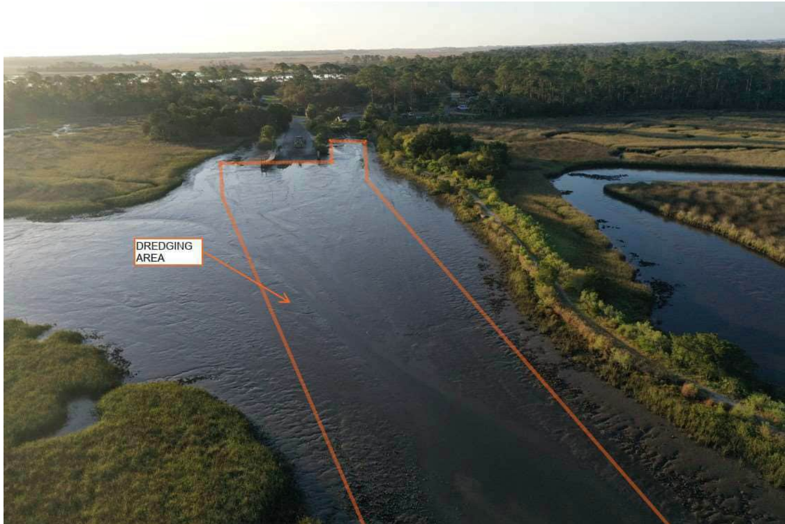
PHOTO 5 – LOOKING SOUTH TOWARD RAMP AND CAMPGROUND. CHANNEL IS COMPLETELY FILLED WITH SEDIMENT AND UNUSABLE FOR BOATERS.
