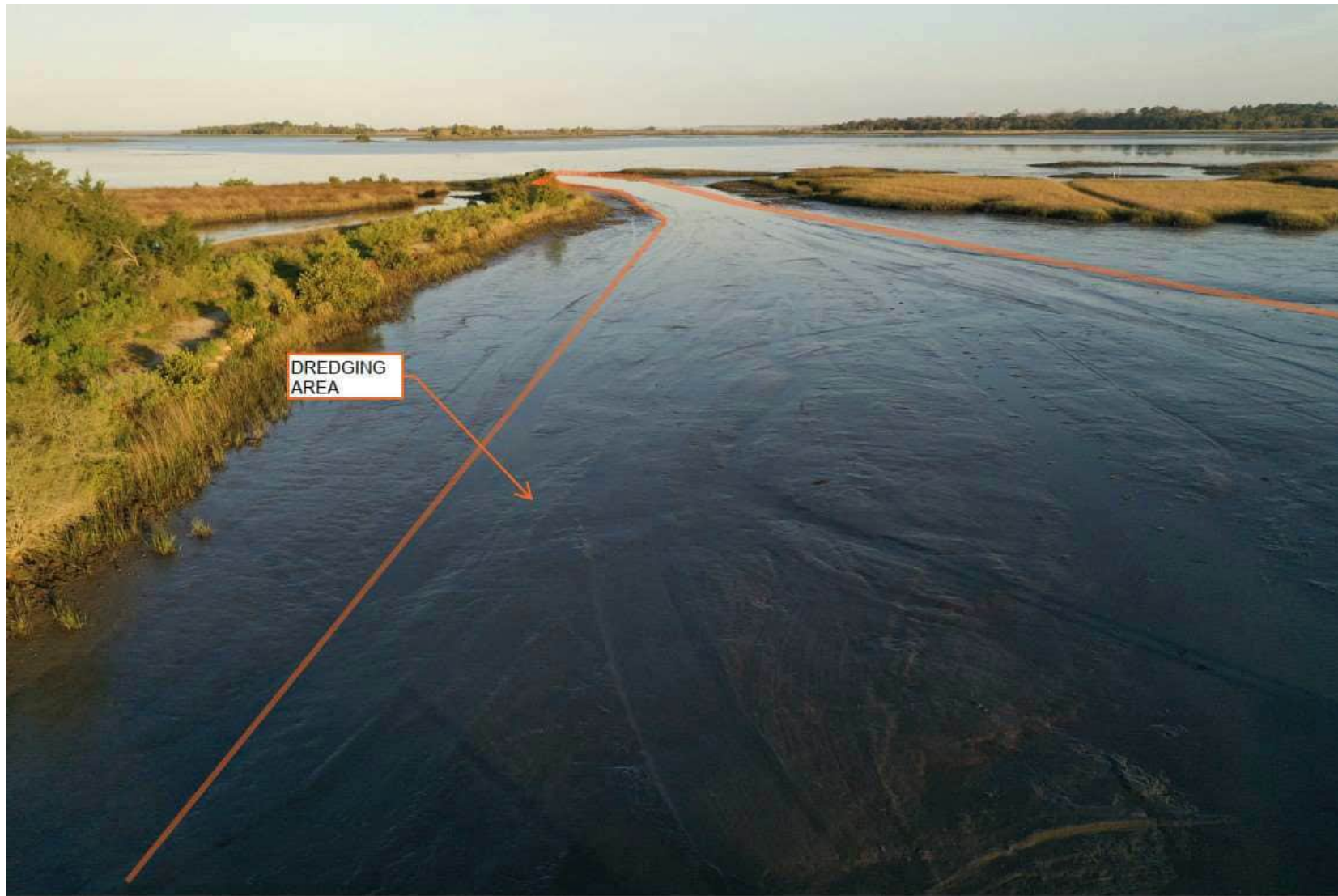
PHOTO 1 – LOOKING NORTHWEST TOWARD MOUTH OF CHANNEL. SEDIMENT LEVELS UP TO 4 FEET DEEP MAKE CHANNEL IMPASSABLE.
