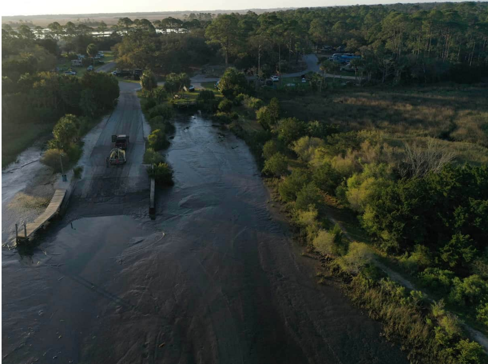
PHOTO 6 – CLOSE UP OF BOAT RAMP LOOKING SOUTHEAST. BOAT RAMP CAN ONLY BE USED BY AIRBOATS EXCEPT AT HIGH TIDE.
