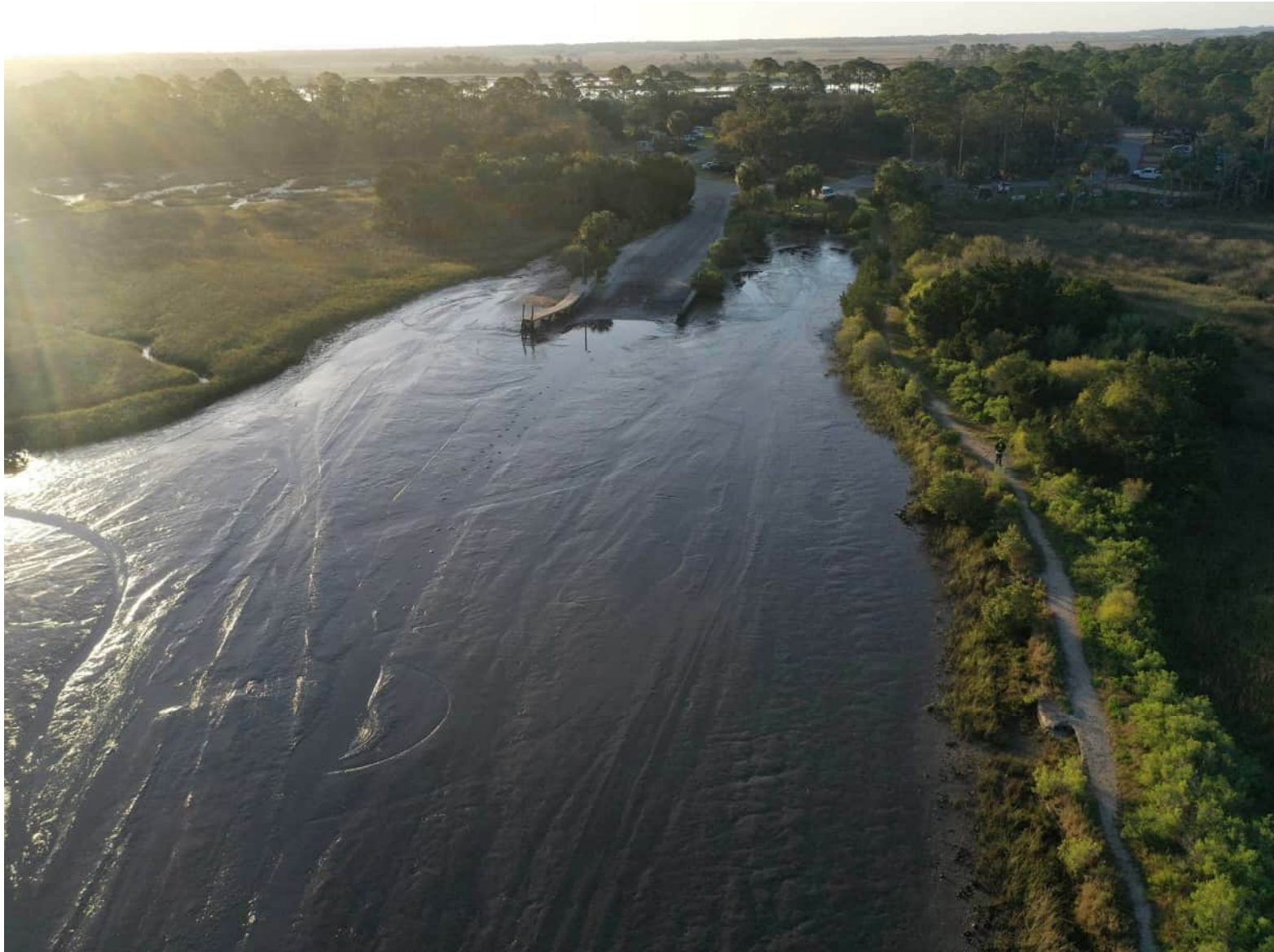
PHOTO 4 – LOOKING SOUTHEAST TOWARD BOAT RAMP. NO DEFINABLE BOAT CHANNEL DUE TO SEDIMENT BUILDUP SINCE LAST DREDGING IN 1990.
