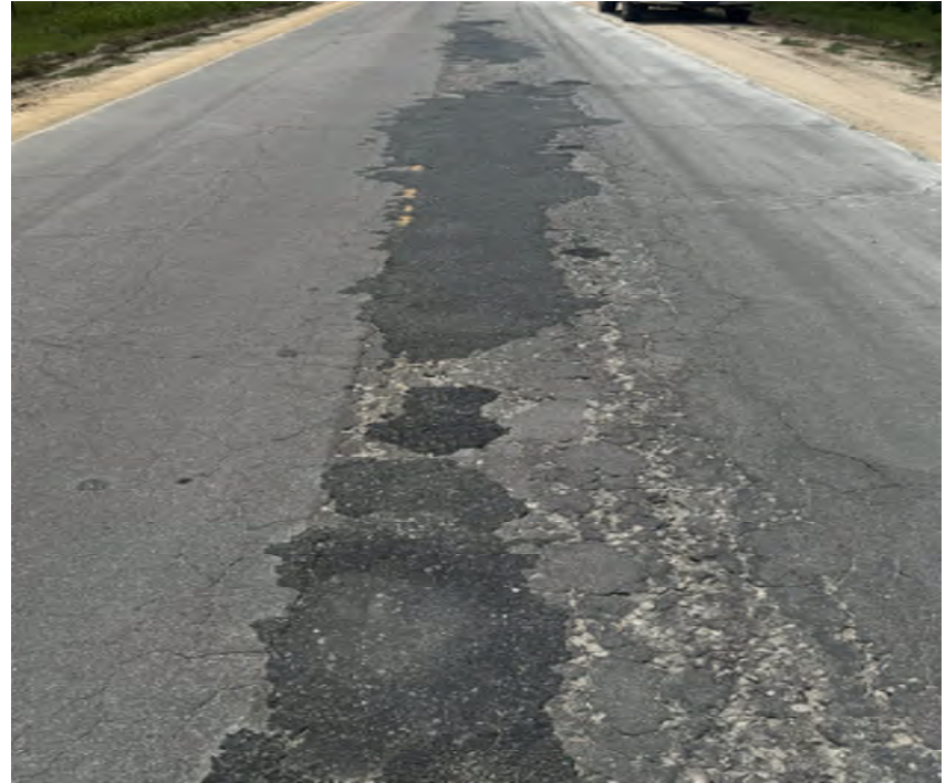
1267+00 to 1268+00 – Asphalt Patches/Potholes
