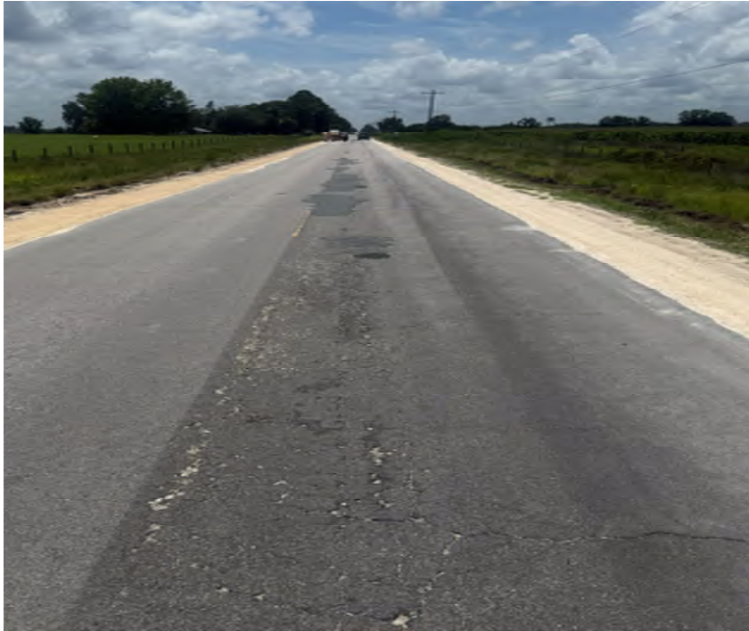
1267+00 to 1268+00 – Asphalt Patches/Potholes
