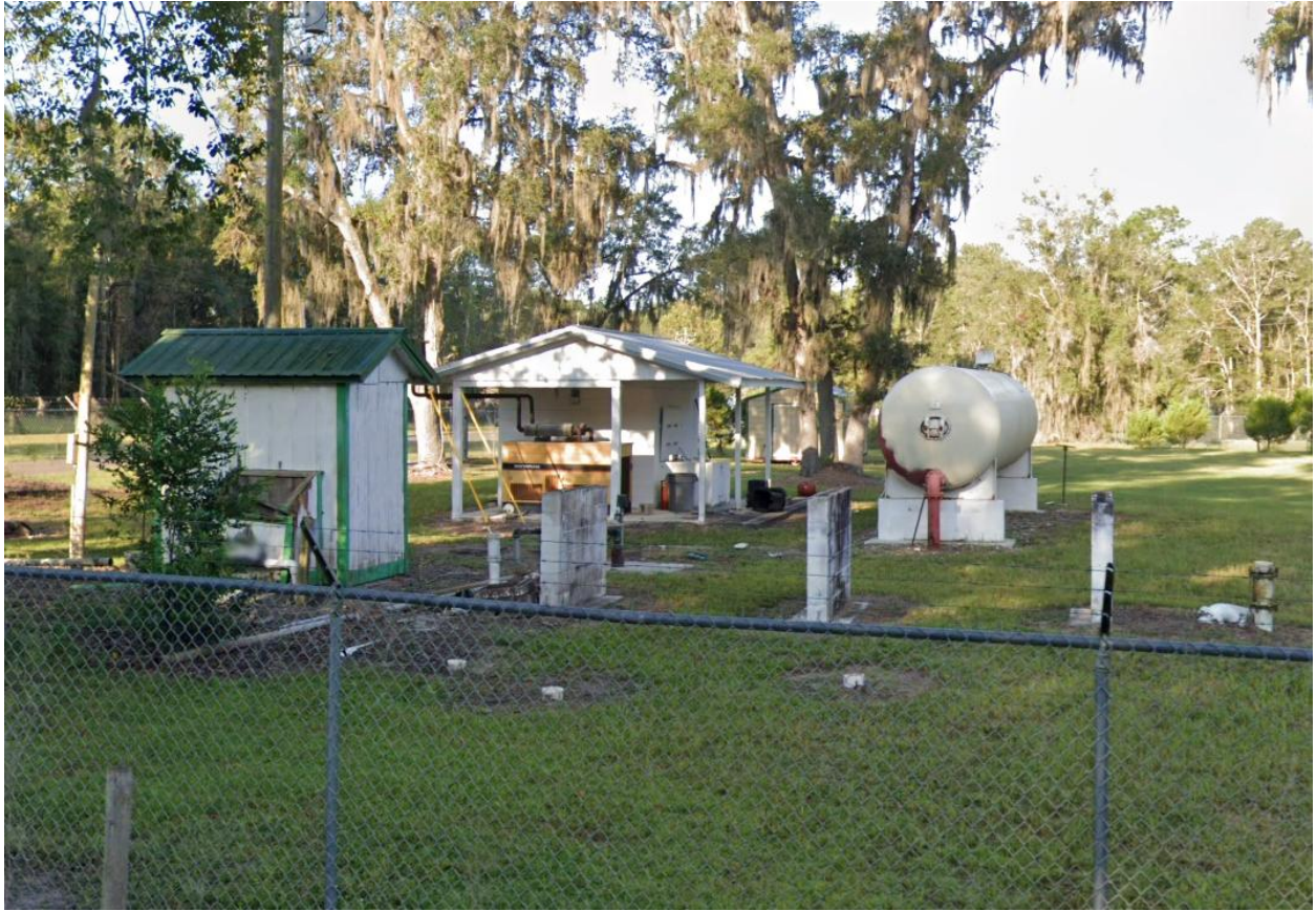
Figure 7: University Oaks WTP looking to the West
