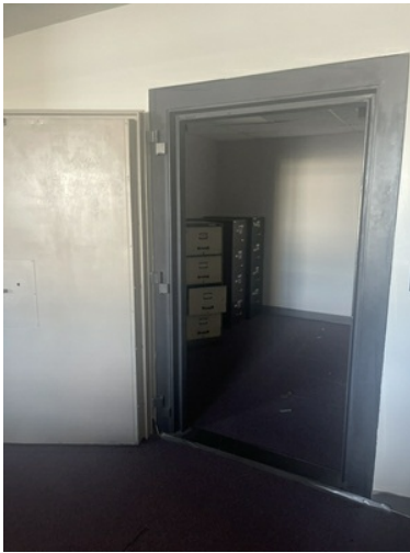
Interior View - Vault/Storage
