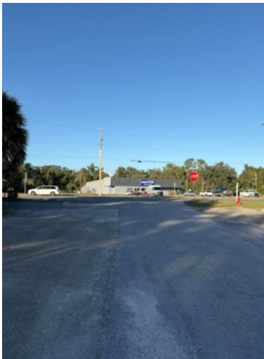
View North Along Oak Street
