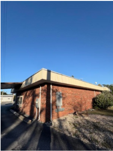
Exterior View - Subject Property
