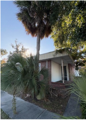
Exterior View - Subject Property
