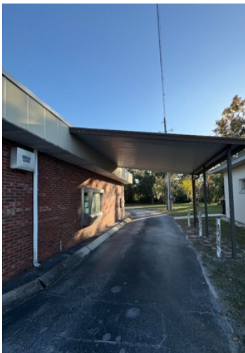
Interior View - Canopy
