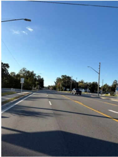
View West Along East Hathaway Avenue
