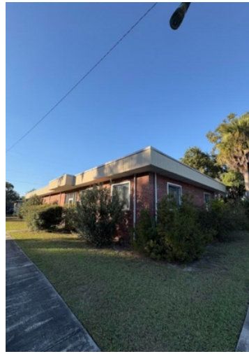
Exterior View - Subject Property
