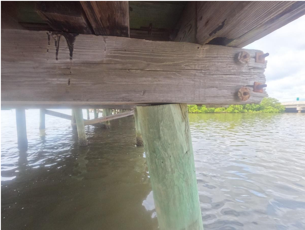
Photo 13: Typical CCA treated pile. Note pile not fully engaged with pile cap and large void in end of stringer (upper right). See below images.
