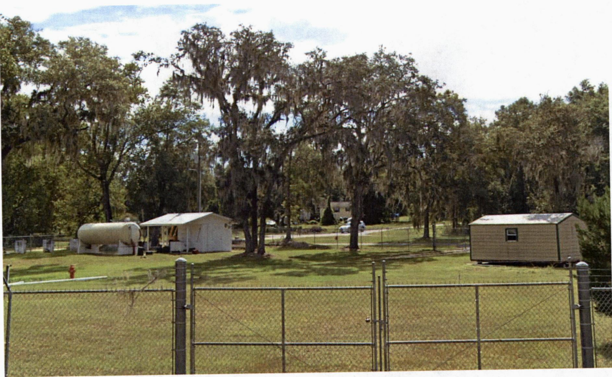
Figure 8: University Oaks WTP looking to the East
