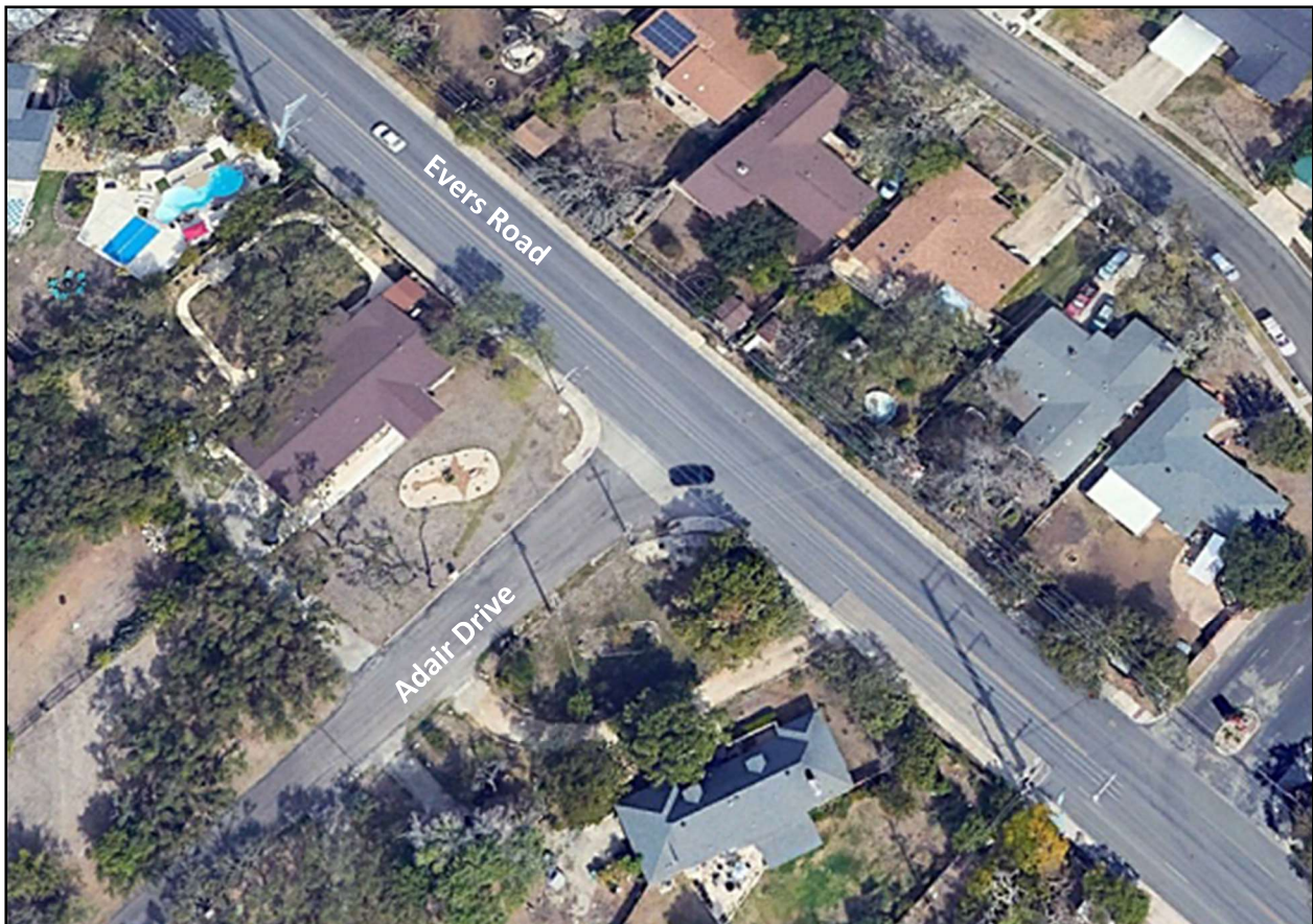
Figure 1. Evers Road and Adair Drive Intersection
