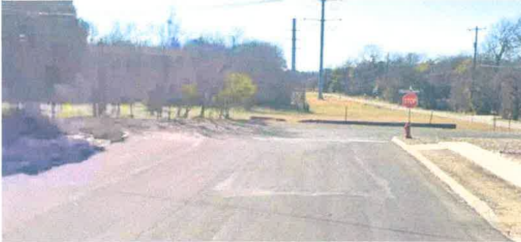
Figure 3. Seneca Drive, westbound at William Rancher Road
