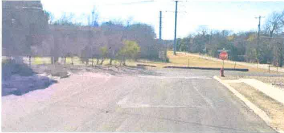
Figure 3. Seneca Drive, westbound at William Rancher Road
