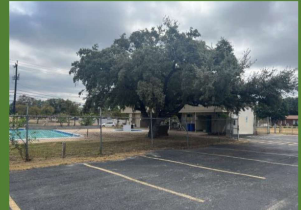
2024 condition of the pool building
