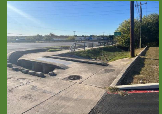
Adjacent trail connecting to the street
