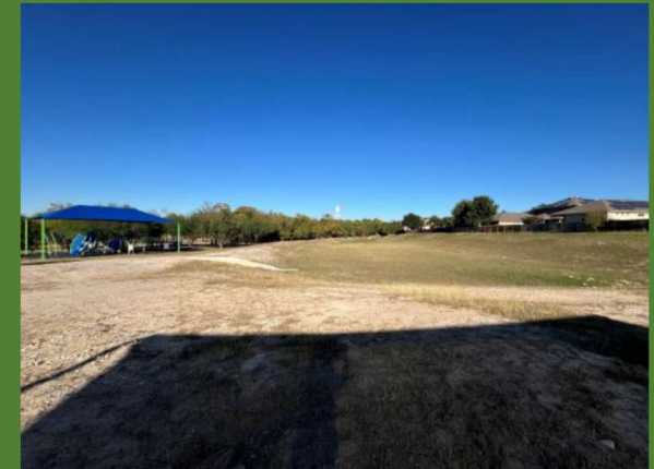
Multi-use detention pond with a playing field area
