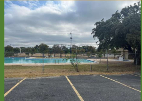
2024 condition of the pool
