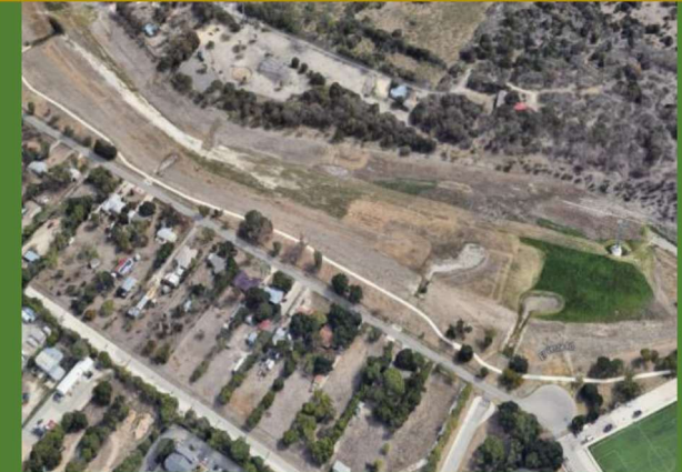
Overview of the Huebner Creek Greenway
