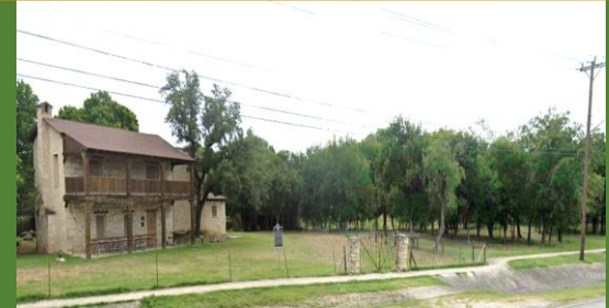
Onion House, historical building at Huebner Onion Park, a desired regional park
