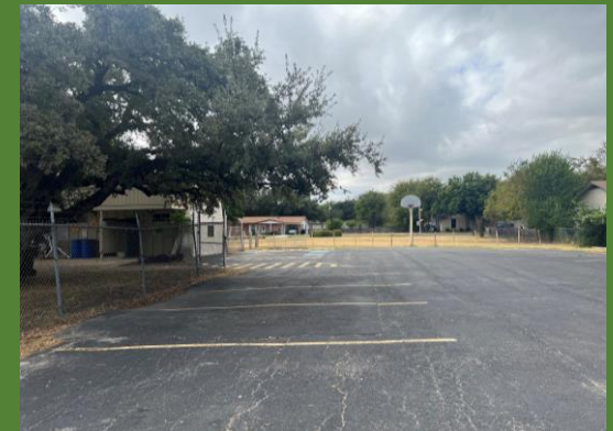
Leon Valley pool parking lot and vacant lot
