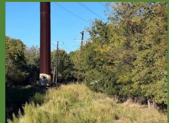
A potential trail along the utility lines
