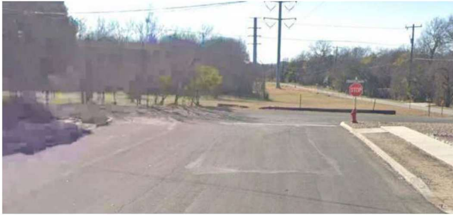
Figure 3. Seneca Drive, westbound at William Rancher Road
