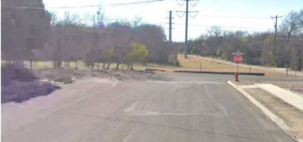
Figure 3. Seneca Drive, westbound at William Rancher Road
