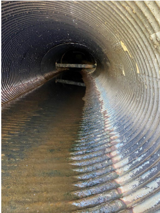
View of interior of pipe. Corrosion evident at interface of baseflow (water), air and steel pipe. An obstruction (gasline) is evident in this photograph.
