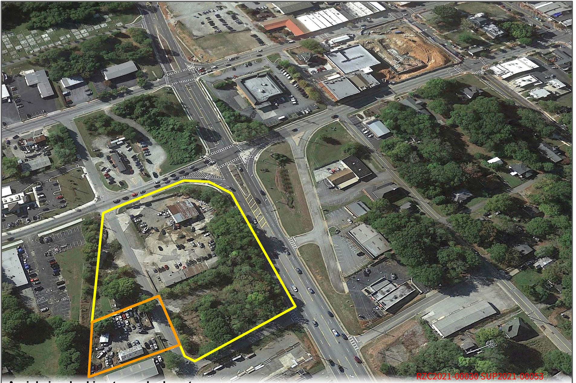
Aerial view looking towards downtown.
