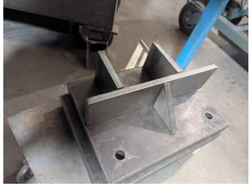
Image of footings with materials prior to welding
