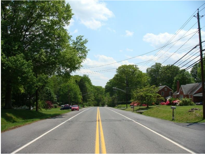
Figure 6: Brooklyn Bridge Road, with shoulders striped for parking
