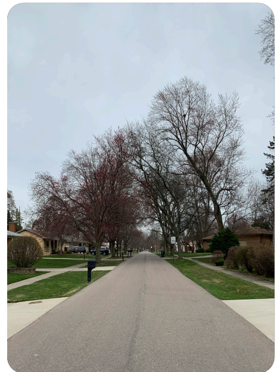
Residential City Street in Lathrup Village (Giffels Webster)
