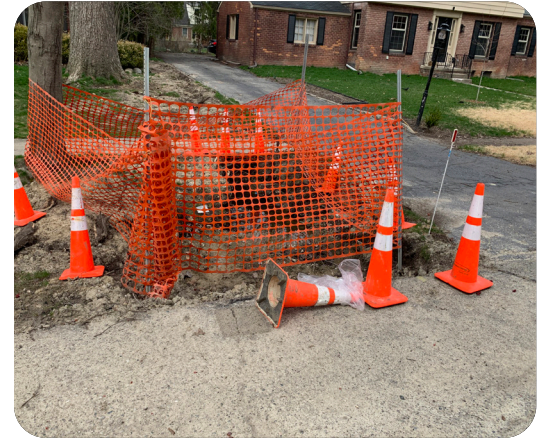
Drainage ditch repair (Giffels Webster)
