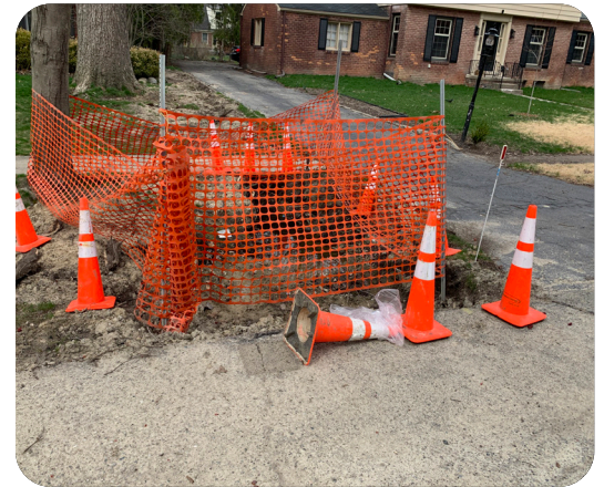
Drainage ditch repair (Giffels Webster, 2020)
