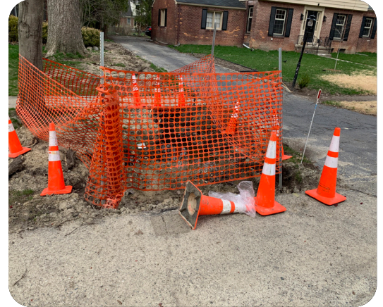
Drainage ditch repair (Giffels Webster)
