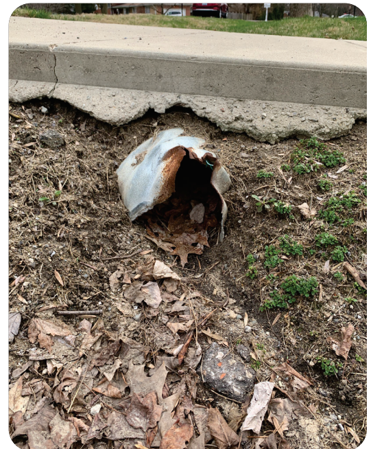
Damaged storm sewer culvert (Giffels Webster, 2020)
