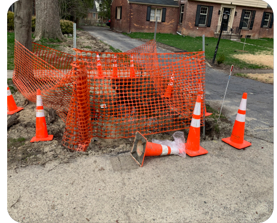
Drainage ditch repair (Giffels Webster)
