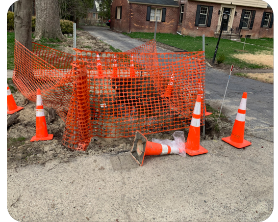
Drainage ditch repair (Giffels Webster)
