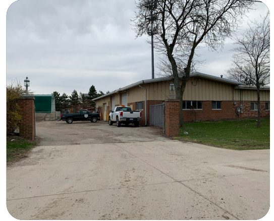
Lathrup Village DPS yard (Giffels Webster)
