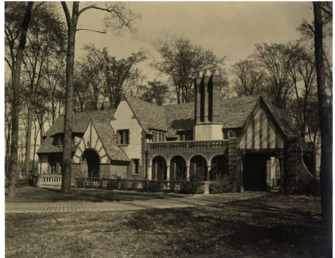
Above: Historic photo of the house (source: Detroit Public Library Digital Images)
