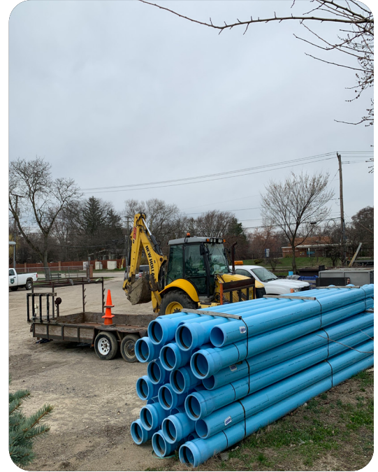
Lathrup Village DPS yard (Giffels Webster, 2020)
