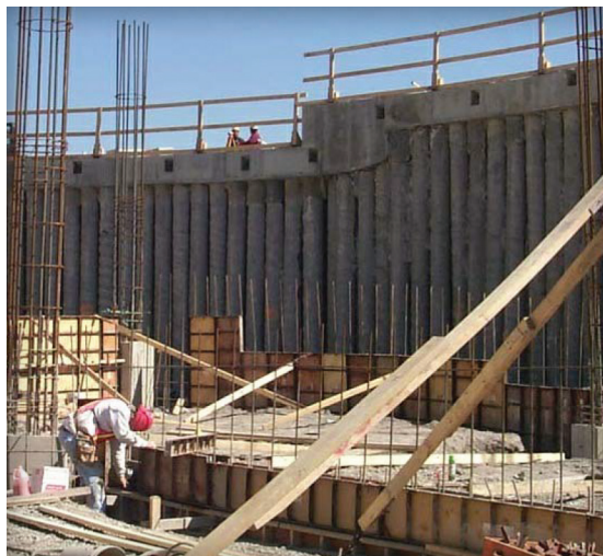
Earth Retention Wall Design and Construction
