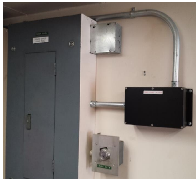
Photo 11. This energy monitor installed next to the control panel tracks energy consumption on up to 12 EVSE and provides access to the data through an online interface.
