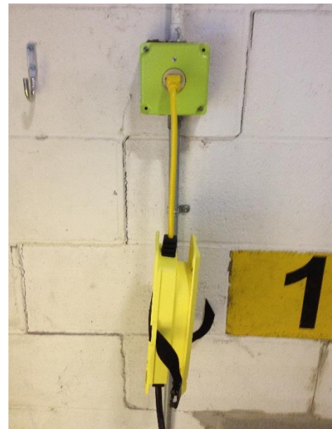
Photo 4. This cordset is hanging from an outlet which may cause strain on the cordset and outlet.
