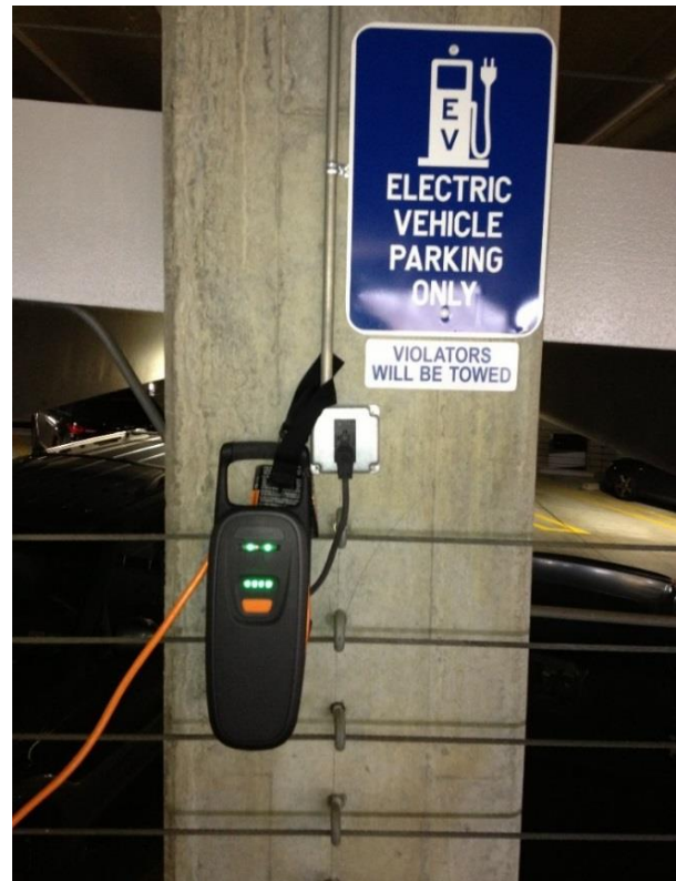
Photo 6. One of many highly visible Level 1 charging stations at Coca-Cola. The driver straps the cordset to the electrical conduit so there is no strain on the plug and outlet. The parking spot is well marked with an Electric Vehicle Parking Only sign.
