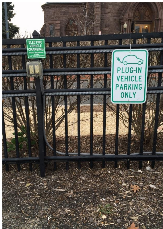
Photo 1. This Level 1 outlet is available for electric vehicle charging at the U.S. Senate parking lot.
