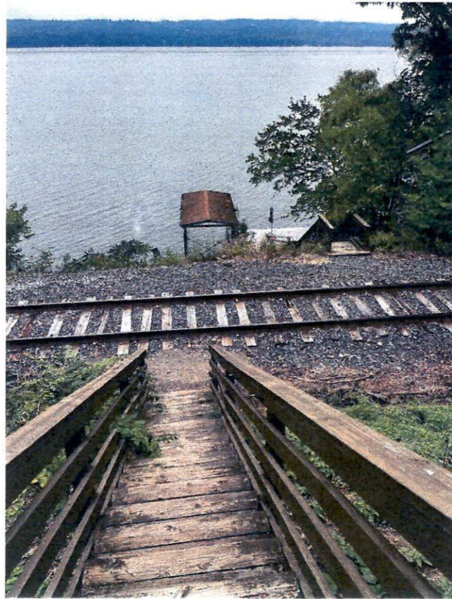
Looking down upper stairway to RR Crossing, Lower Access Stairs, and Lake View of 281 Bill George Rd.
