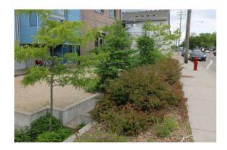
Stormwater management with tree trenches, bioretention planters and stormwater planters
