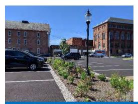
**Description:** Shallow stormwater controls that utilize vegetation and engineered filter media to capture, treat, and infiltrate stormwater runoff into the underlying soils.
