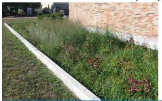
**Description:** Passive filtration system to manage and treat small to moderate volumes of stormwater runoff from adjacent impervious surfaces. The system consists of an inflow component, a shallow ponding area over a planted soil bed, mulch layer, stone drainage layer, plantings and an overflow mechanism to convey larger rain events to the storm drain system.
