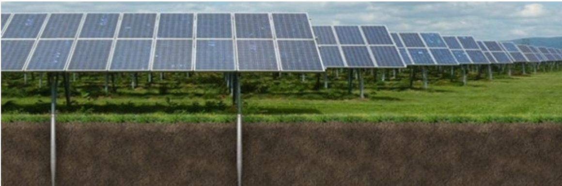
Figure 3b. Supporting Structure Overview
