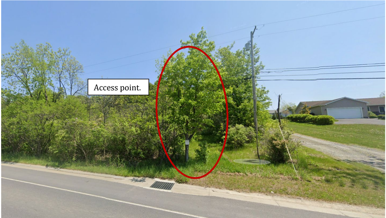
Figure 1b. Access Point
