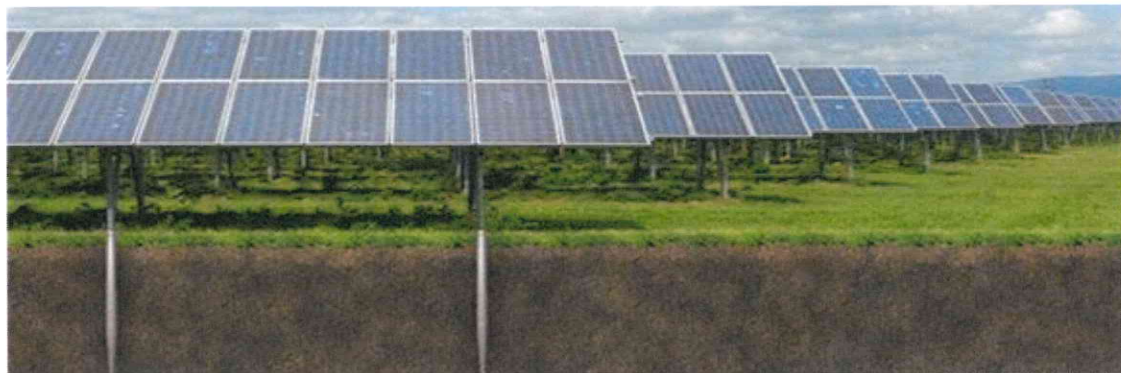
Figure 3b. Supporting Structure Overview
