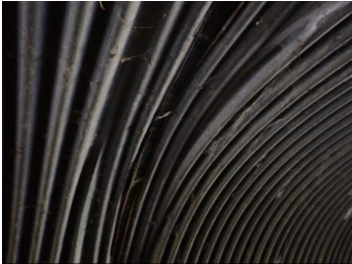
DIFFERENTIAL SETTLEMENT IN MIDDLE SEAM, NORTH SIDE
