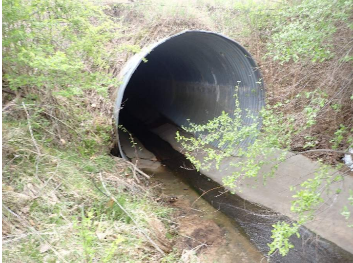
WEST ELEVATION, INLET, NO VISIBLE DEFLECTION
