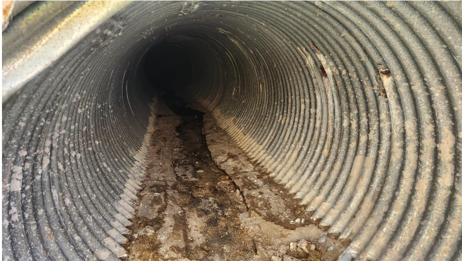
Photo #1 – Existing CMP Pipe under 4H Road
