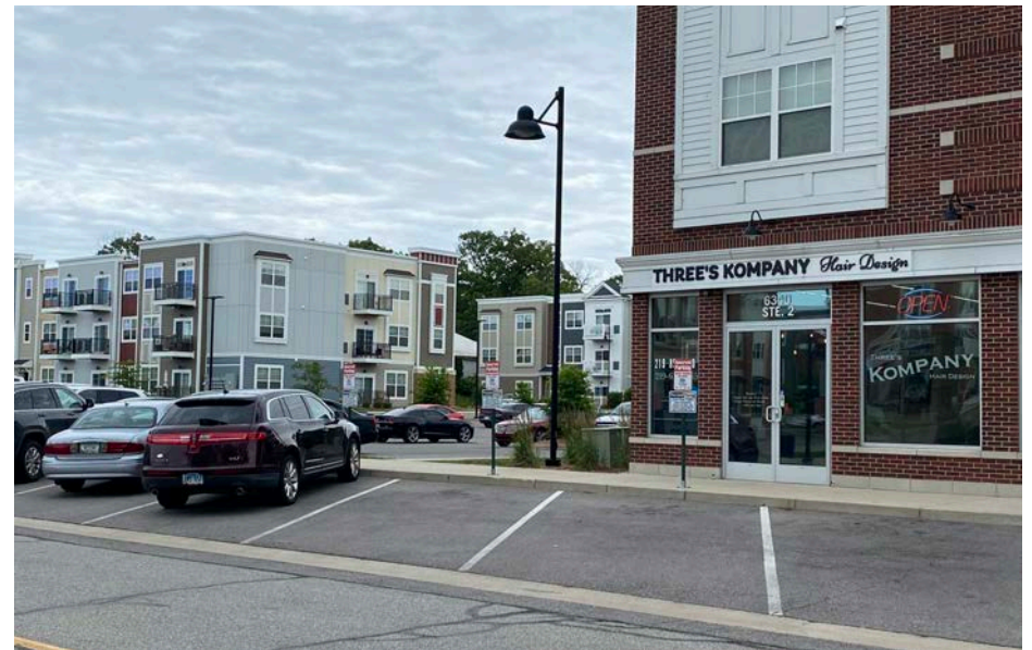
Founders Square, Portage, Indiana. A new town center in a suburb along a major street corridor, similar in many ways to the Towne Center site.
