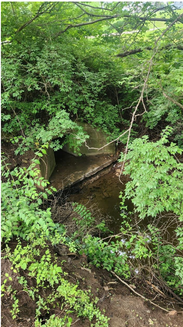
Plunge Pool at Box Culvert Outfall
