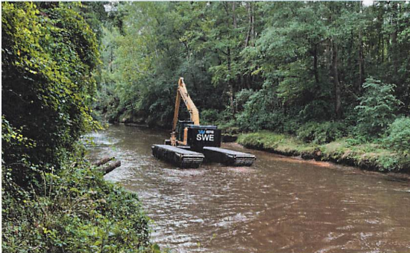
Before & After: Back Swamp Stream Debris Removal
