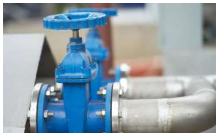
Gate Valve Installation for Isolation $5,000,000
