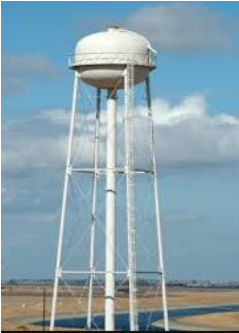
MULTI-LEG 100,000 GALLON WATER TANK
