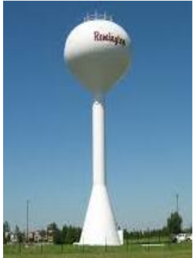
SPHERIOD 100,000 GALLON WATER TANK
